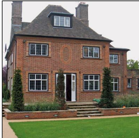
A two store extension carefully detailed to respect the main building
