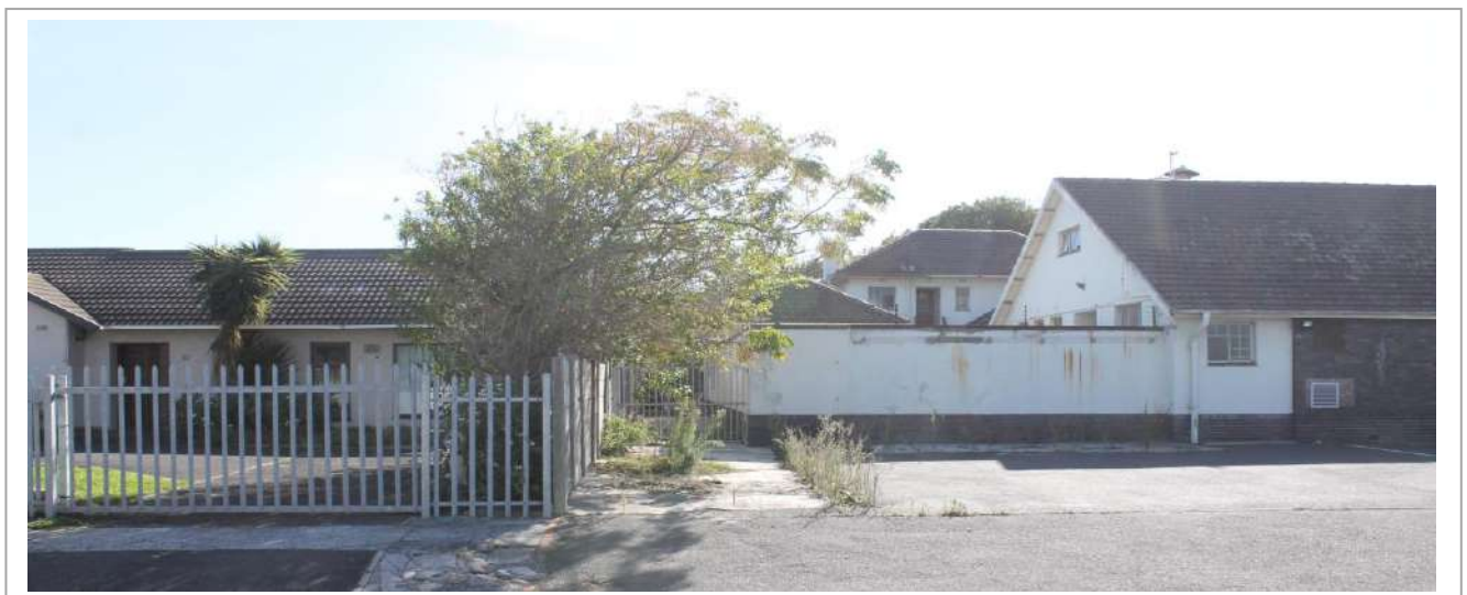
Photo 2: Shows the boundary condition between Erf 2643 and 3133 Pinelands
