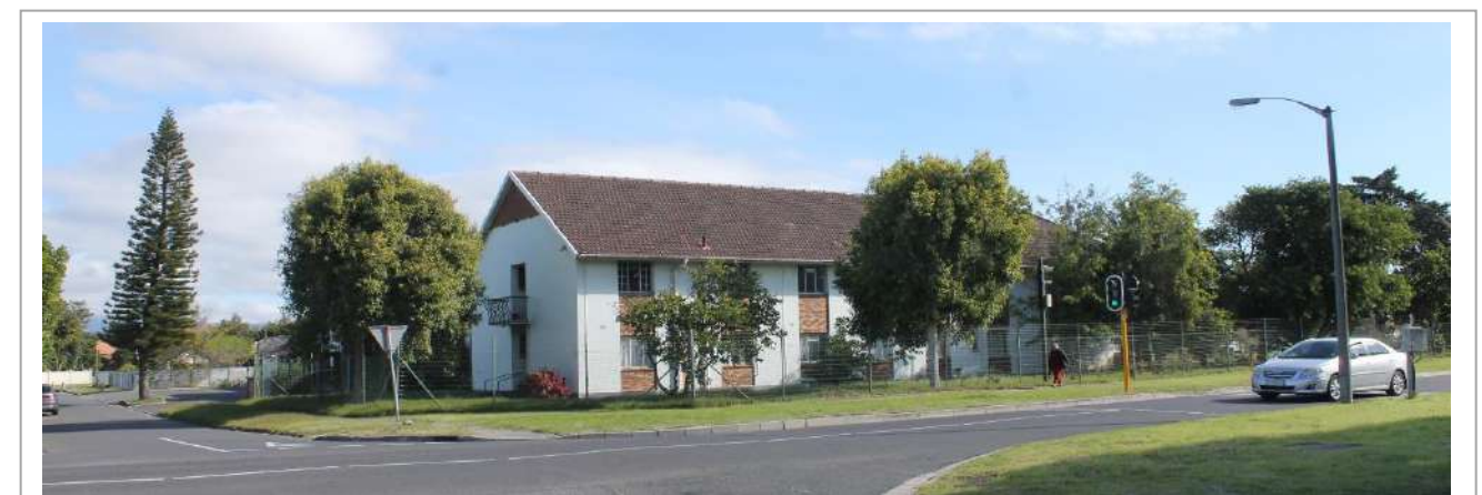
Photo 3: The Howard Drive façade and edge that is located approximately 8,74m from the road reserve
