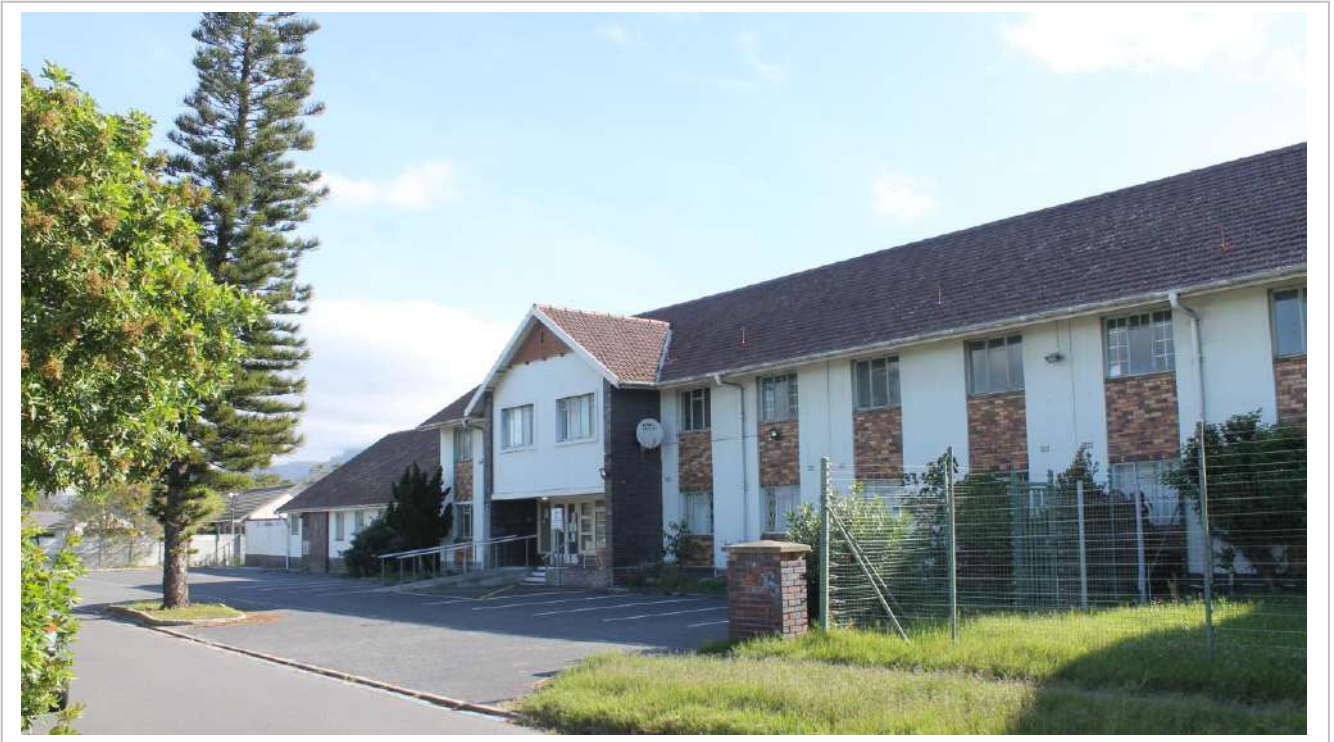
Photo 1: SAWAS façade facing Cedar Road
